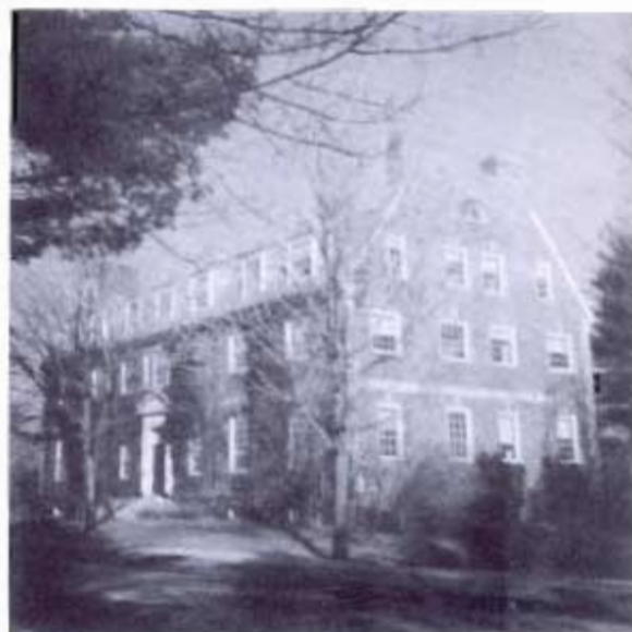
Lyon Hall — Classrooms and Offices
